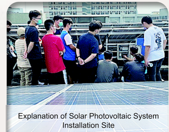
Installation Explanation and Implementation of Solar Photovoltaic Modules
