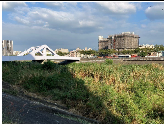
Current Status of the Test Points
