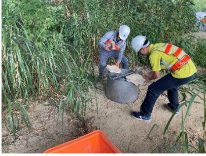
Installation of Double-Ring Infiltrimeters
